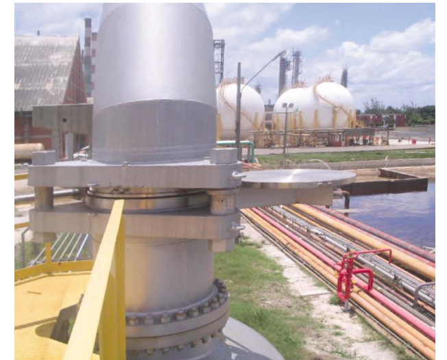
Cam-Set® DN 500 (20"), ASME 150# with spectacle plate support
